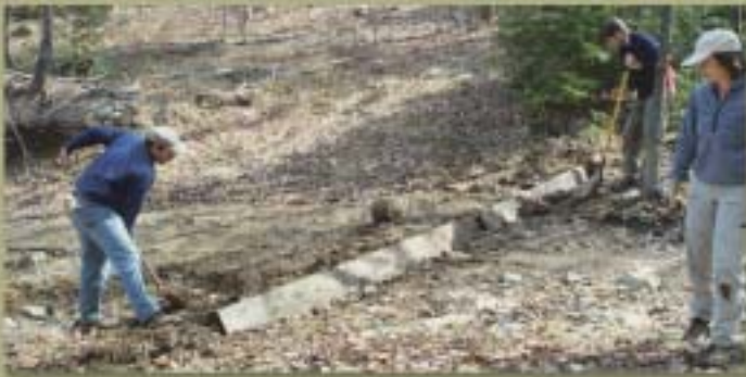
LGLC volunteers Mandy and Rocco Giampaolo and LGLC conservation assistant Chris Krahling install waterbars at our Gull Bay Preserve.
